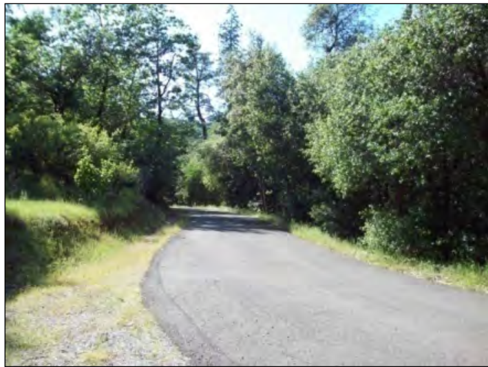
Bailey Road. Note dense brush and trees to pavement edge.
