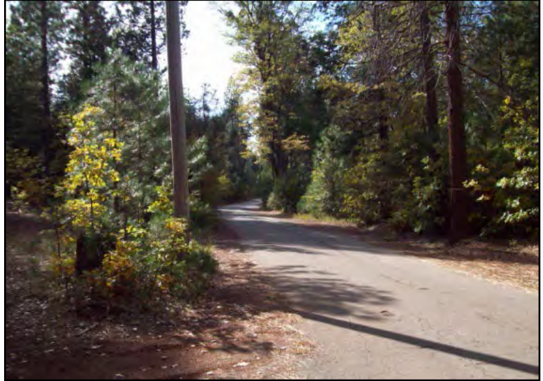
Shingletown Ridge Road. Note trees and brush up to asphalt edge.
