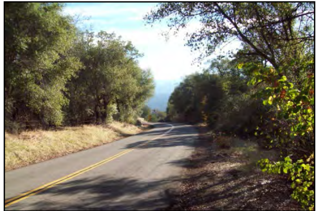
Black Butte Road. Note dense trees and brush near asphalt edge.
