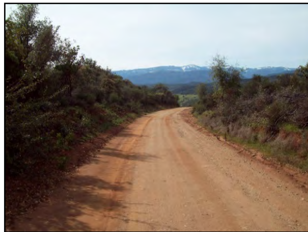
Bully Choop Road. Note thick vegetation to sides of road
