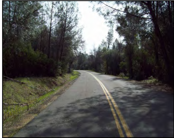
Rainbow Lake Road – note heavy tree and brush growth to edge of road.
