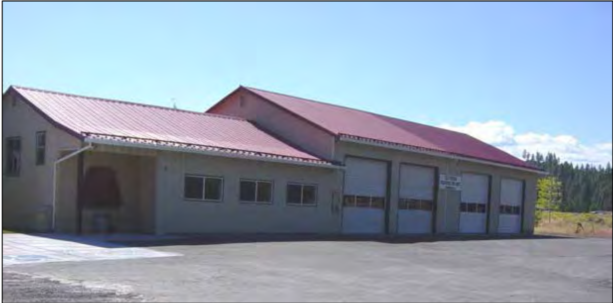
Old Station volunteer firehouse
