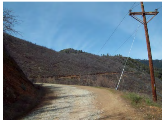
Summit Gulch. Ridgetop along which fuelbreak would be constructed
